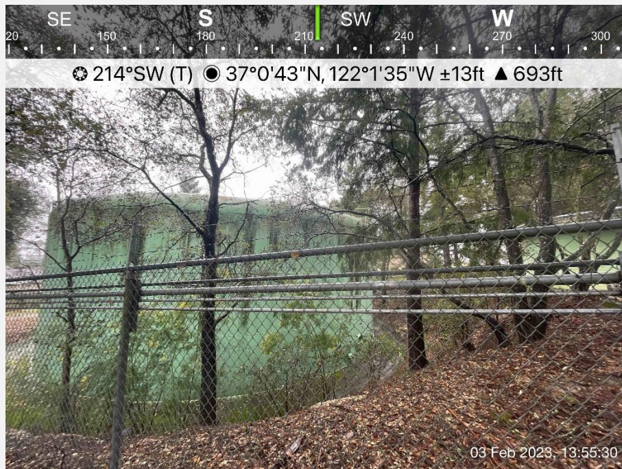
Photo Number 6. Pasatiempo tank site.
