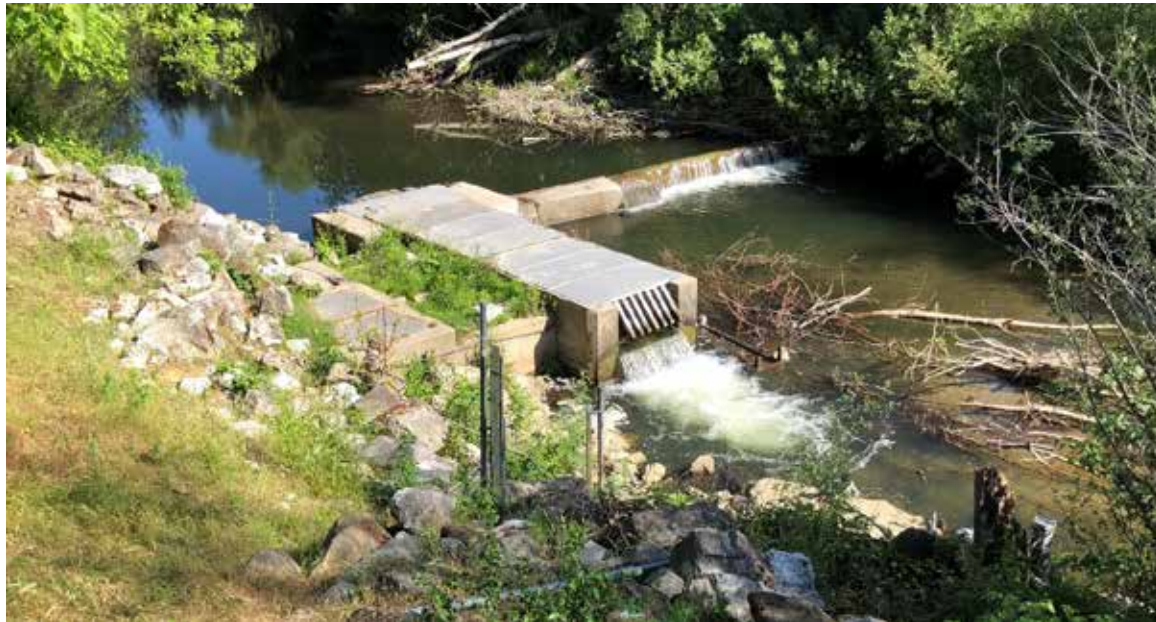
Exhibit 5. Tait Diversion, overview showing the 1983 intake in the foreground and the remaining section of the original concrete diversion dam stretching across the San Lorenzo, view looking north (IMG_0175).
