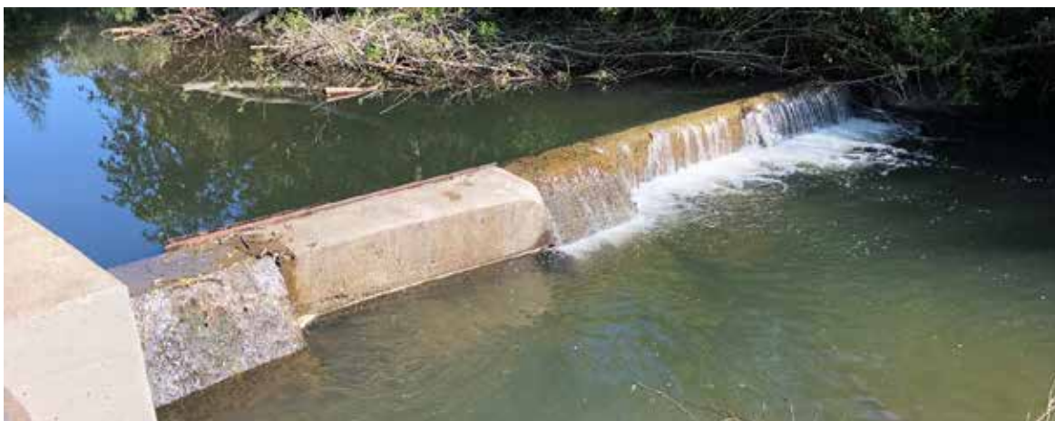
Exhibit 6. Tait Diversion, remaining section of the original concrete diversion dam, view looking north (IMG_0165).
