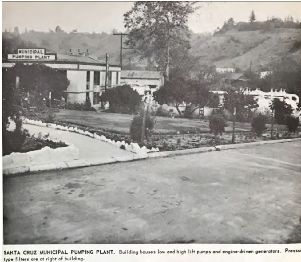
Figure 10. The Municipal Pumping Plant as it appeared in 1956 (Brown and Dunlap 1956: 18).
