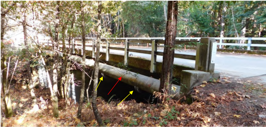
Exhibit 11. View of the NCP (red arrow) showing the existing hangars (yellow arrows) supporting the pipeline as it crosses beneath the Newell Creek Access Road Bridge, view looking northeast (DSCN6306)
