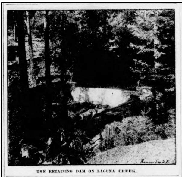
Figure 6. The earliest known photograph of the Laguna Creek Masonry Dam published in the Santa Cruz Surf in 1892 ( Santa Cruz Surf 1892: 2).
