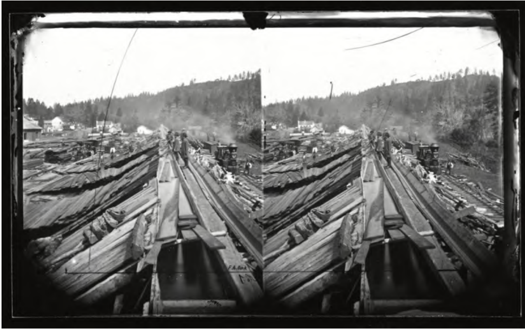
Figure 3. An early photograph of the Felton Flume (center) alongside the narrow gauge Santa Cruz and Felton Railroad (engine and tracks at right) (University of California, Santa Cruz Special Collections).
