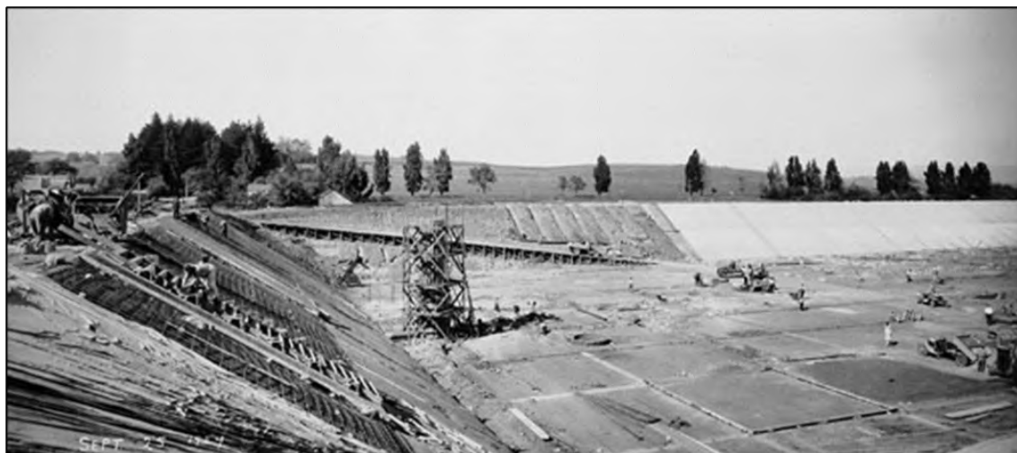
Figure 8. Construction of the Bay Street Reservoir in 1924 (SCPL 1924).
