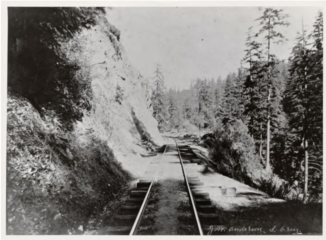
Figure 4. A photograph showing the expansion of either the Santa Cruz and Felton Railroad or the Felton and Pescadero railroad from narrow to broad-gauge in the proximity of Felton, c. 1905 (University of California, Santa Cruz Special Collections).
