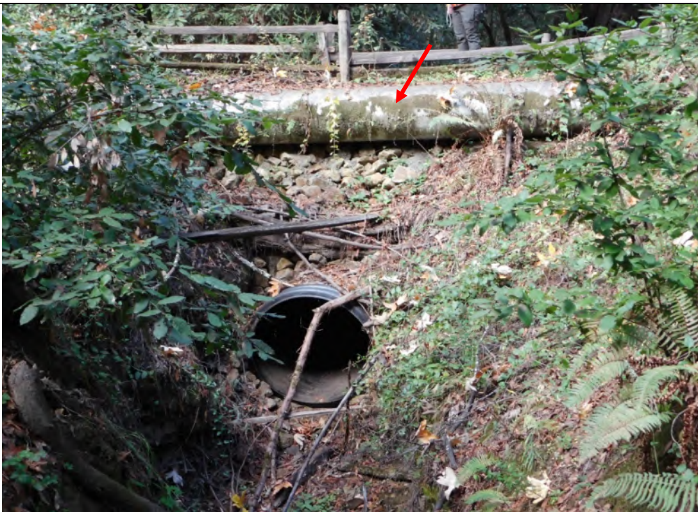
Exhibit 10. View of one of the points where a segment of the NCP is visible (red arrow) as it crosses a culvert under Pipeline Road within Henry Cowell State Redwood Park (DSCN6723)
