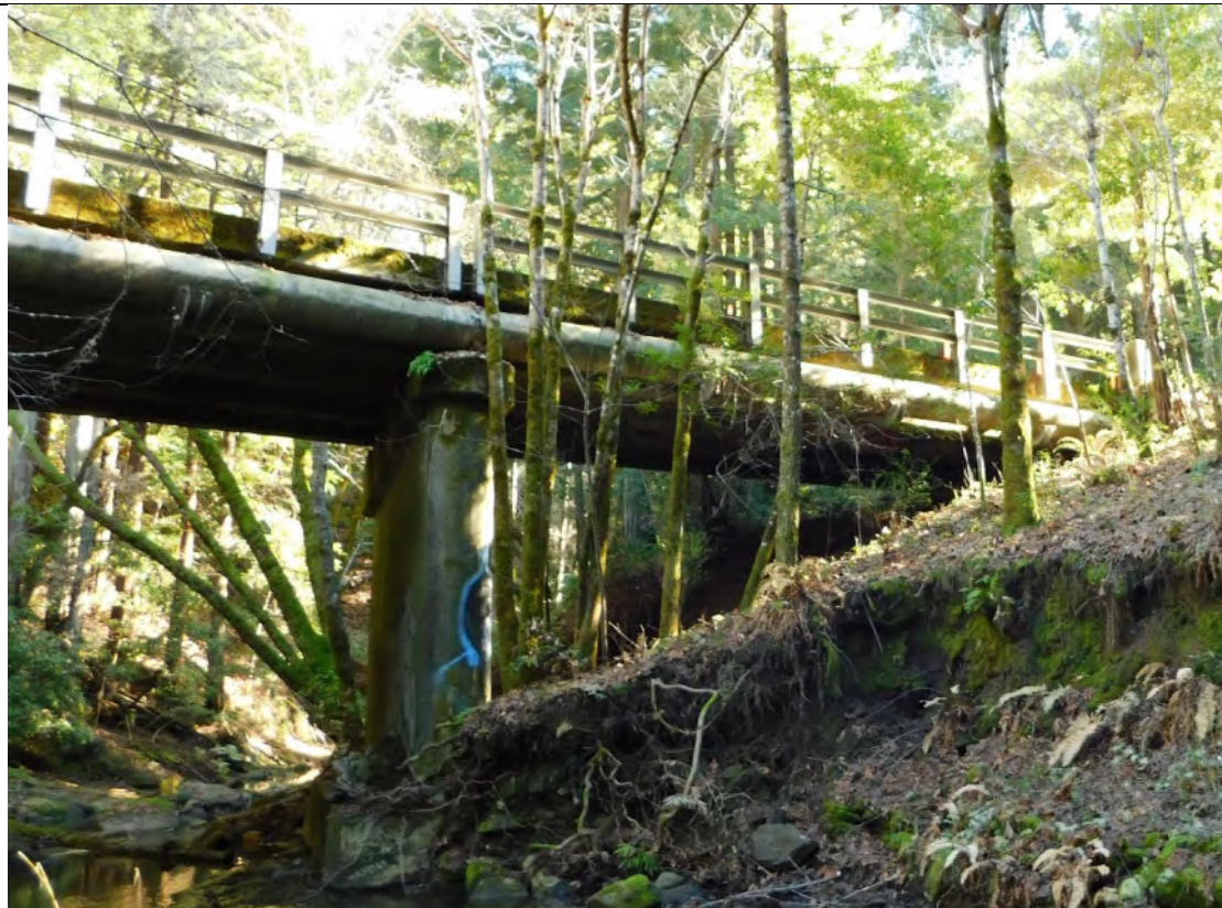
Exhibit 12. View of the NCP as it crosses beneath the Newell Creek Access Road Bridge, view looking southeast (DSCN2812)
