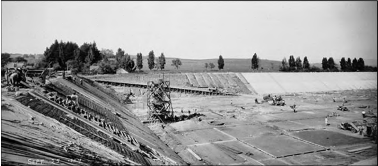
Exhibit 6. Construction of the Bay Street Reservoir in 1924 (SCPL 1924).
