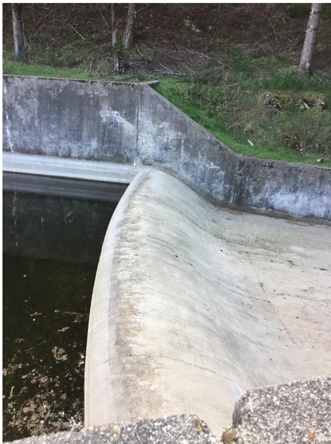
Figure 12. Spillway Inlet at Crest, Looking Southeast. February 20, 2018. (IMG0027)
