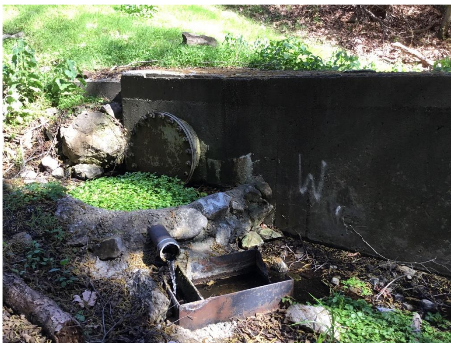
Figure 21. Valve Feature, Weir, and Weir Pool . February 20, 2018. (IMG0113)
