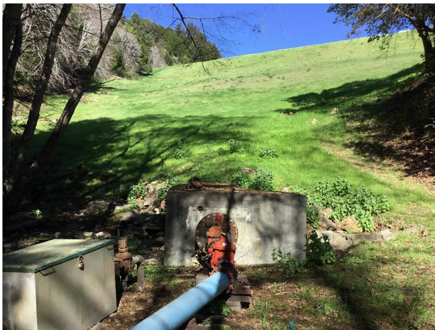
Figure 20. Valve Feature and Concrete Housing, Emerging from Toe of Dam, Looking Northeast. February 20, 2018. (IMG0101)
