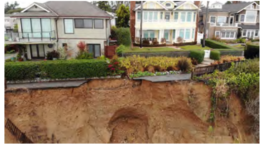
Figure 12b – Grand Avenue Pedestrian Pathway Erosion
