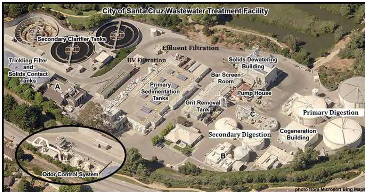
Figure 6-10. City of Santa Cruz Wastewater Treatment Facility
