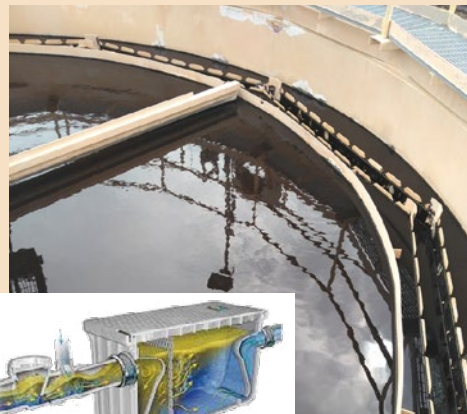
Clean Ocean food manufacturing facilities often install pretreatment clarifiers to reduce solids being discharged to the sanitary sewer. They install cooking air filters and various means of preventing cooking oil and grease from infiltrating wastewater.
