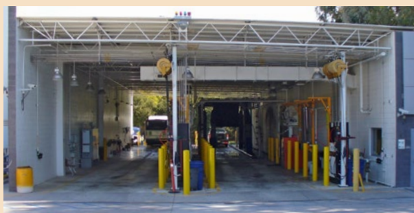
Clean Ocean vehicle service facilities include spill response plans and "looped" covered wash systems to contain wastewater.
