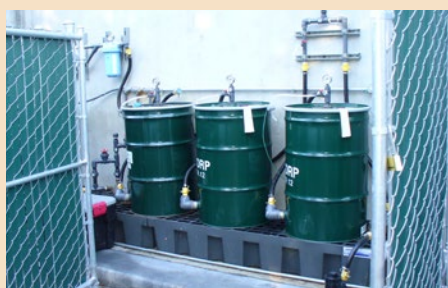
Clean Ocean Business best practices include the installation of carbon filtration systems to clean groundwater before discharge to the sanitary sewer.
