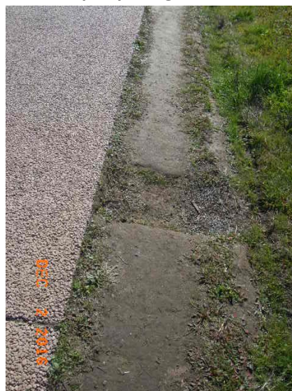
Figure 10. Small gravel drain upslope edge of east-west trail, December 2016
