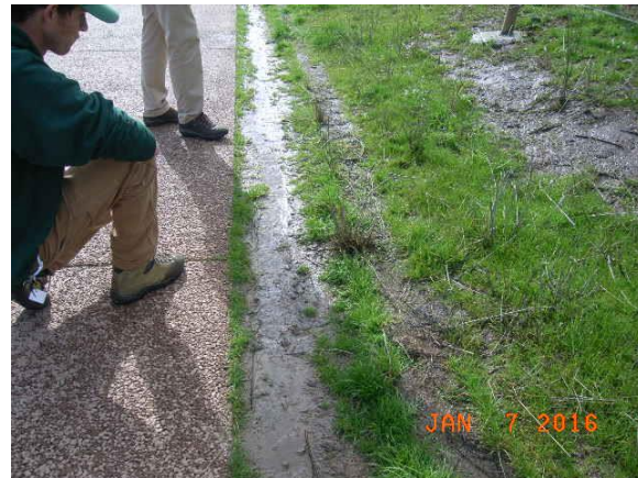
Figure 9. Water collecting on upslope edge of east-west trail, January 2016
