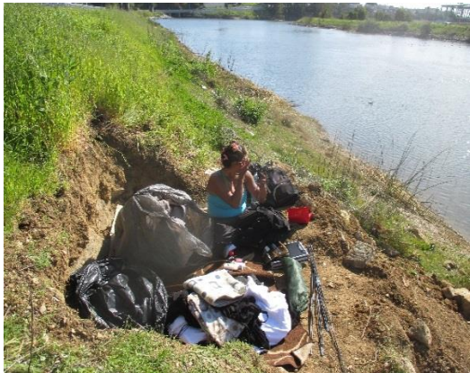
Levee damage caused by illegal camping
