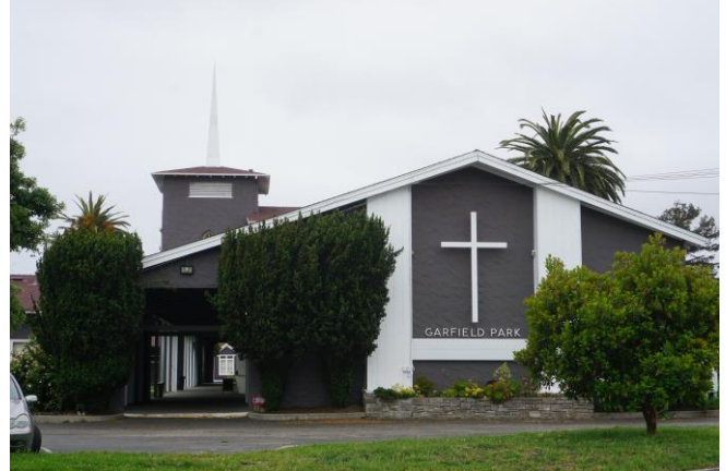
Figure 8: East façade with opening to covered passage.
