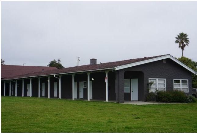
Figure 16: West façade of east wing.
