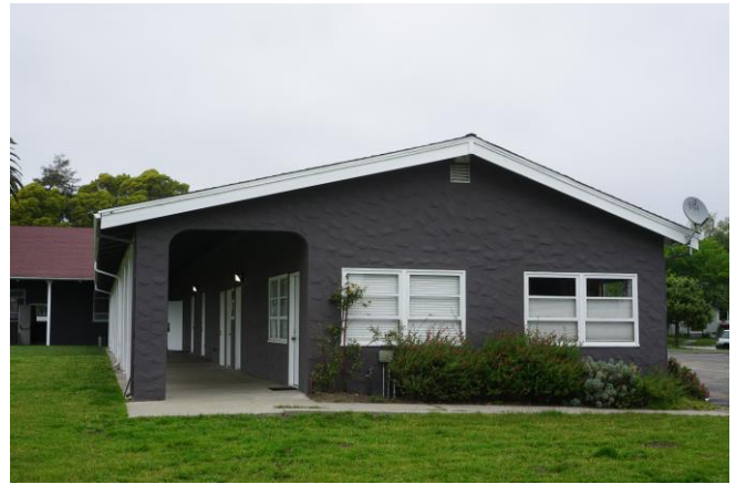
Figure 17: South façade of east wing.
