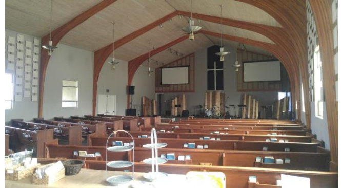
Figure 20: Sanctuary, towards alter.
