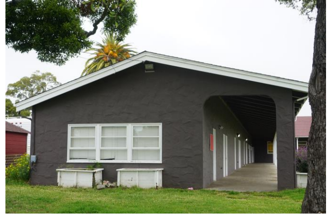
Figure 14: South façade of west wing.
