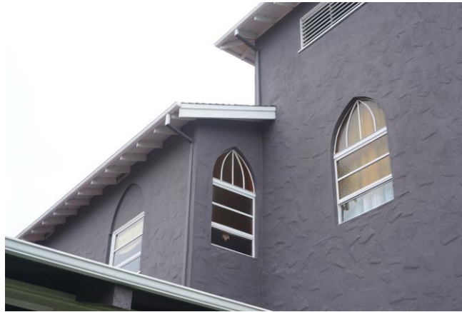
Figure 11: Windows on second story and tower.
