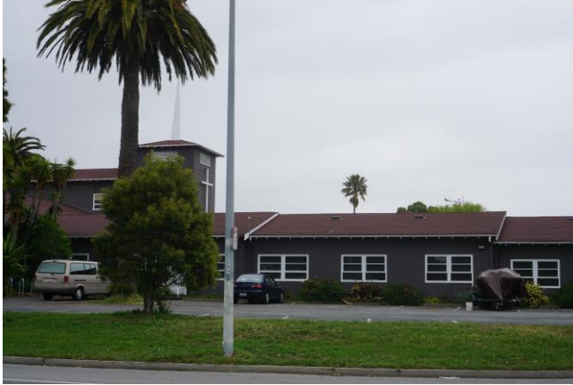
Figure 13: West façade of west wing.
