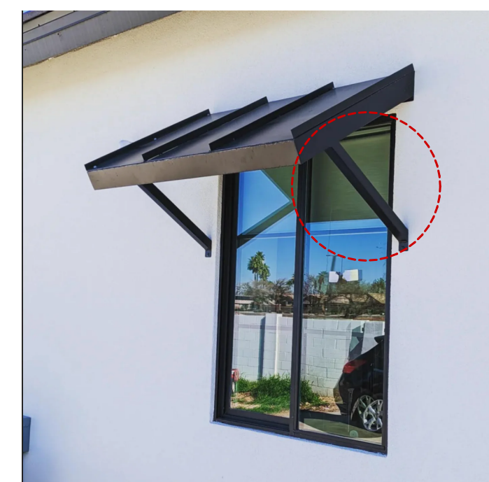
D1-2 NEW POWDER-COATED STEEL BRACKETS
