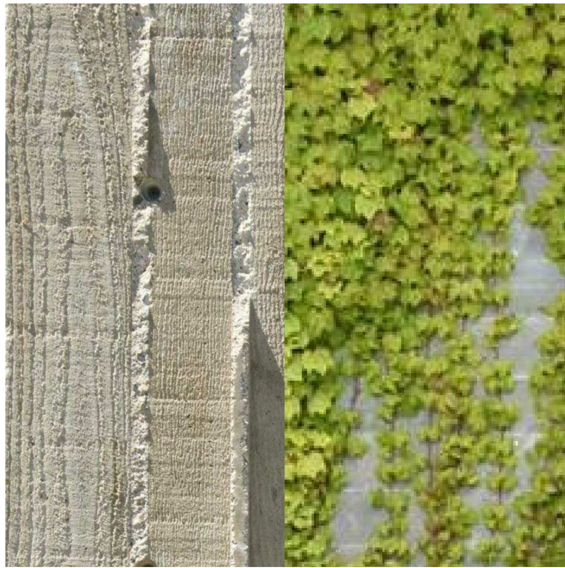
A. BOARD FORM CONCRETE
