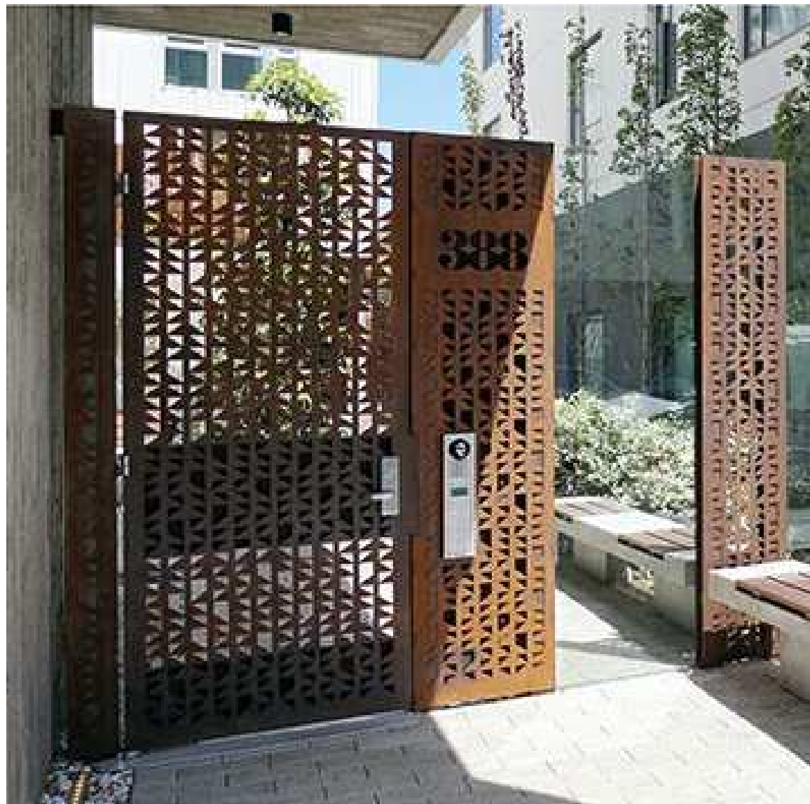
F. PERFORATED METAL SCREEN
