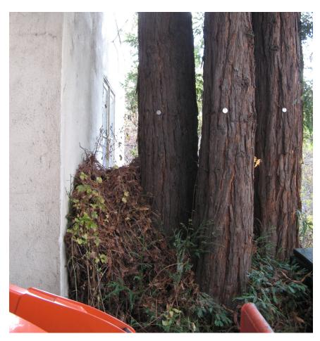
Each of the tree/tree groups grows in proximity to the existing building. Although currently there is no visible damage, there may unseen damage and/or damage may occur in the future from root development.
