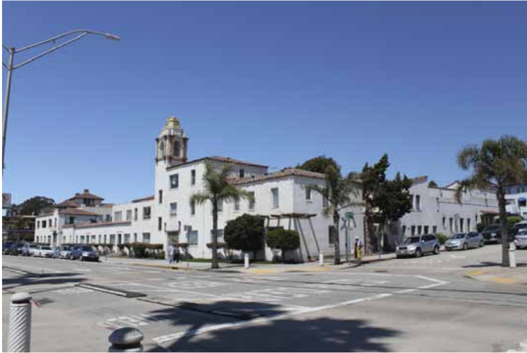
From southeast corner looking west
