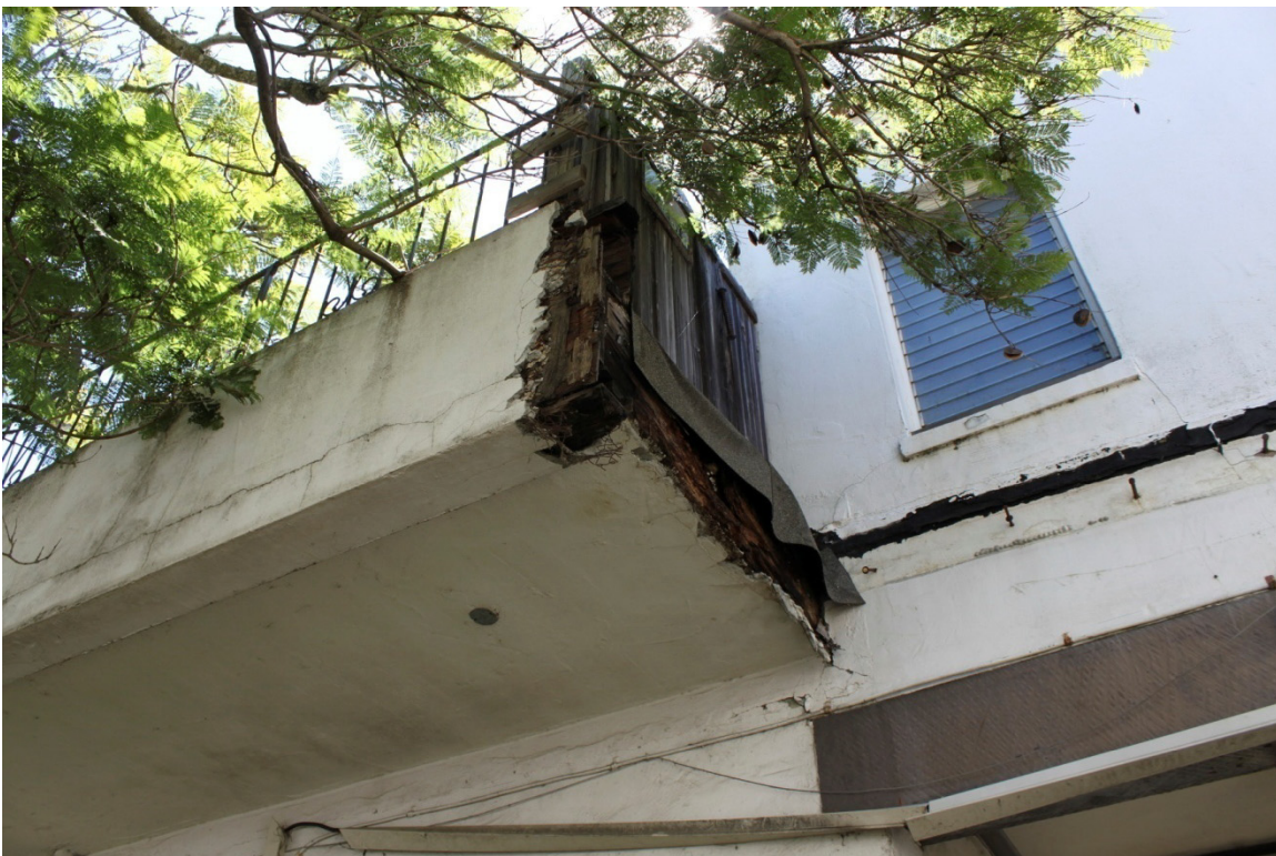
Court of the Mariners, detail; balcony partially removed due to water damage (Architectural Resources Group, July 2013)
