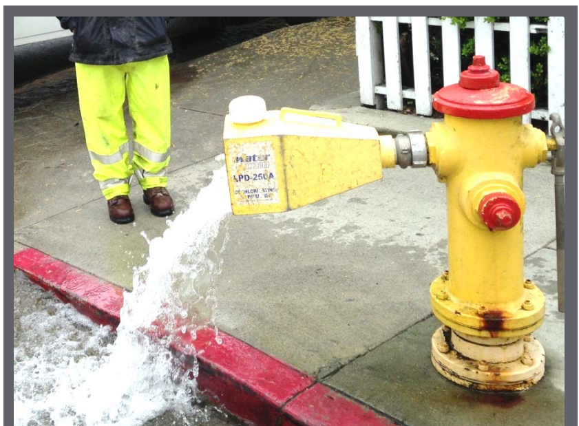
Flushing water lines
