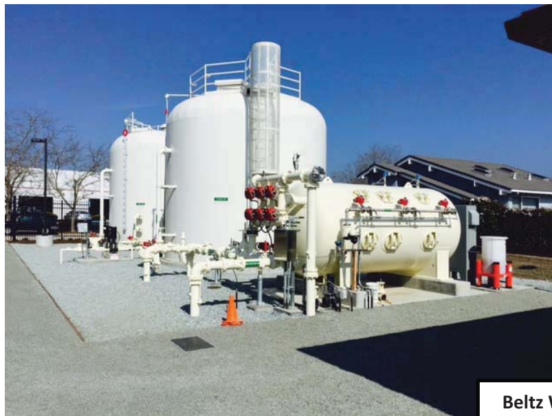
Bay Street Reservoir
