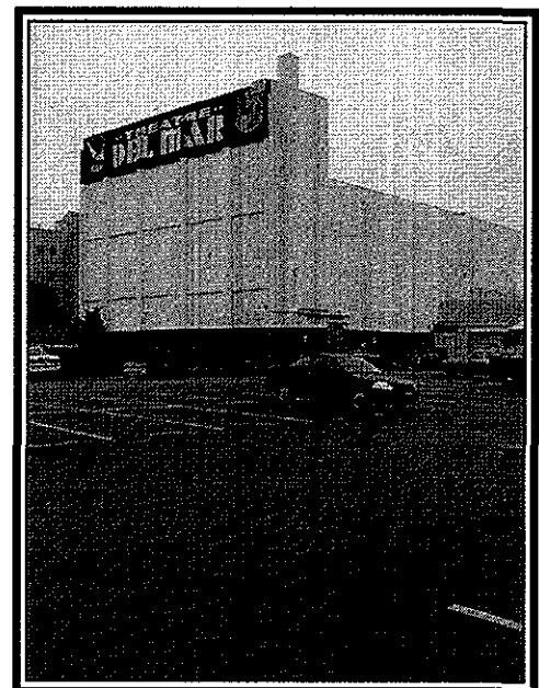
Del Mar Theater, rear view
