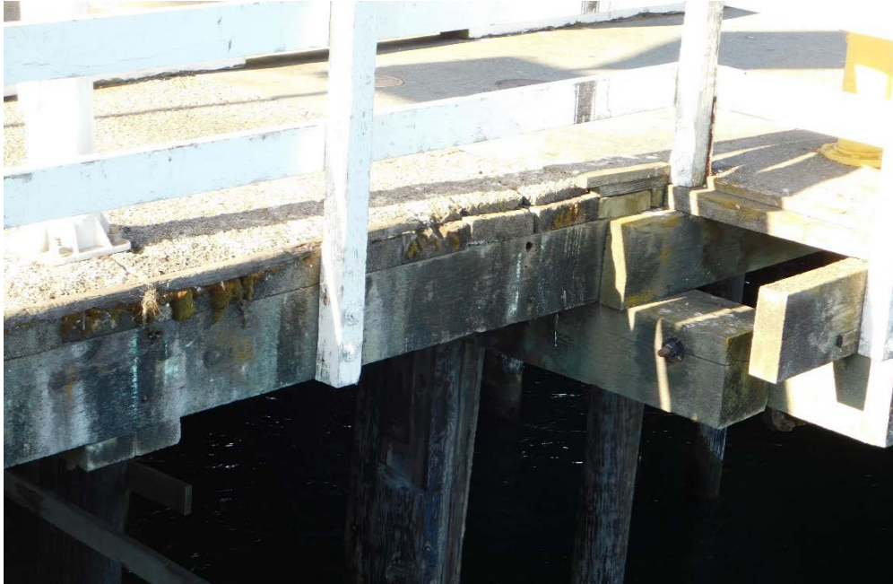
Figure 3. Horizontal stringers supporting layered deck construction (Detail, DSCN 4109)
