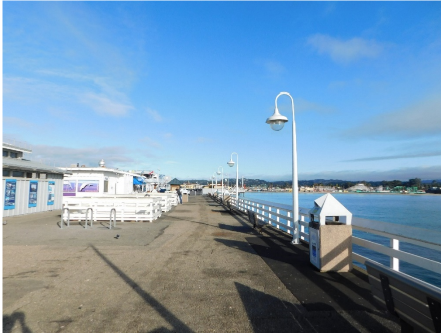
Figure 9. Example of the wooden railing protecting the perimeter of the wharf. Note the fishing access portals at center-left of the photo which are enclosed with the same style wooden railing (View looking north, DSCN 4047)
