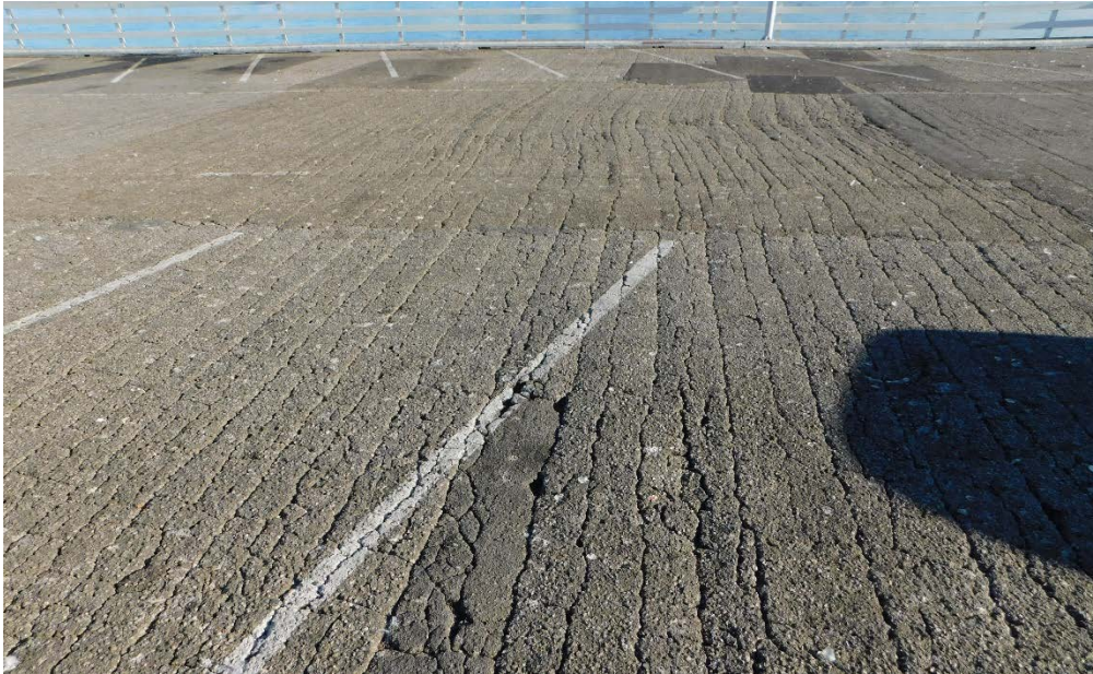
Figure 7. Stress lines in the surface asphalt from the movement of the wharf (View looking east, DSCN 4101)
