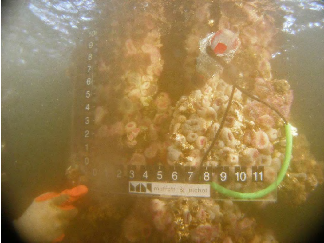
Photo 1-26: Bent 179, Pile 13 – Pile with 90% section loss
