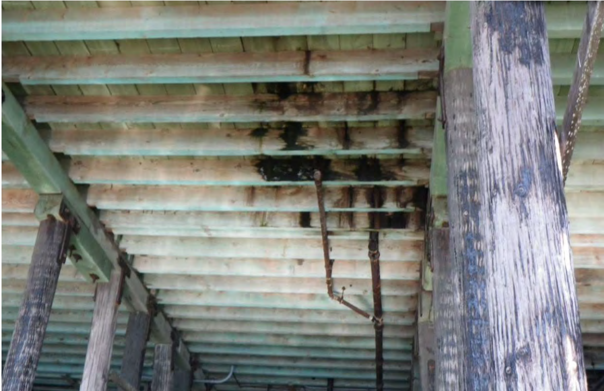
Photo 2-19: Rot from pipe leak Bents 112-113 (west side)
