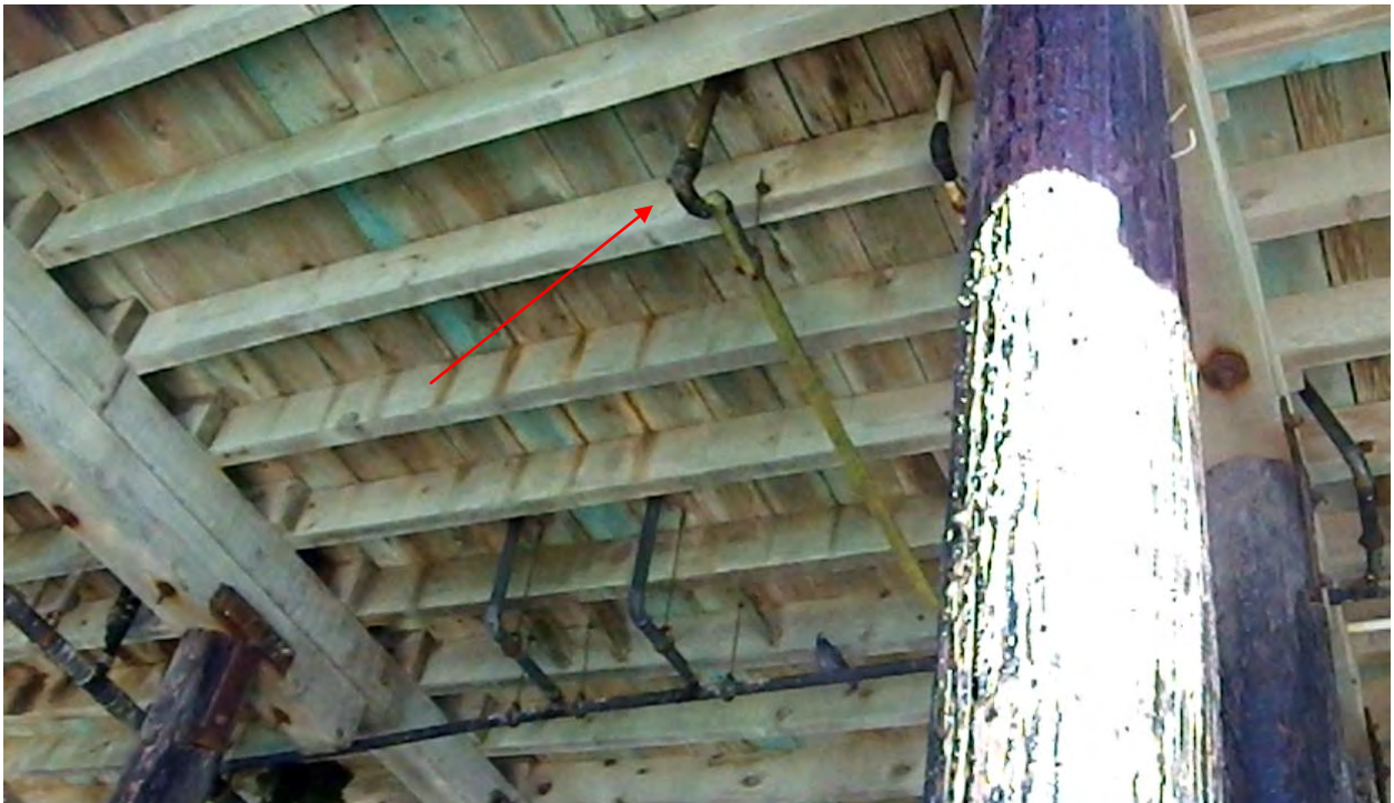
Photo 2-16: Leaking Pipe, between Bent 103-104 west side
