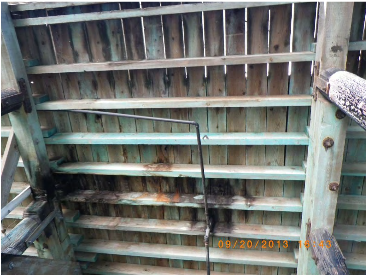
Photo 2-18: Rot between Bent 108-109, west side
