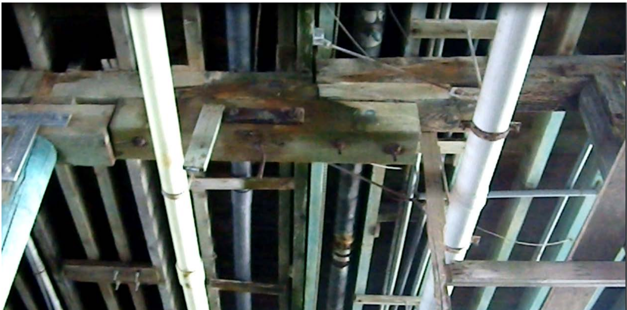
Photo 2-24: Bent 108 - Approx. 13 ft. span & unsupported cap splice.
