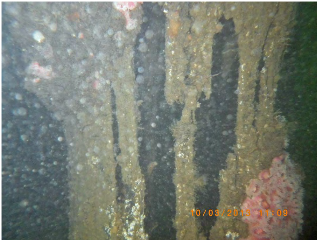
Photo 1-27: Bent 78, Pile 20 – 95% section loss
