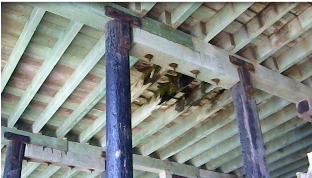
Photo 2-20: Rot between Bent 118-119 (west side)
