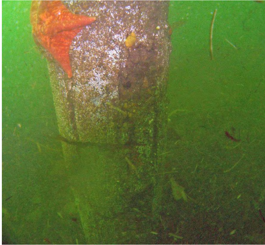
Photo 1-18: Bent 112, Pile 5 - Portion with splits
