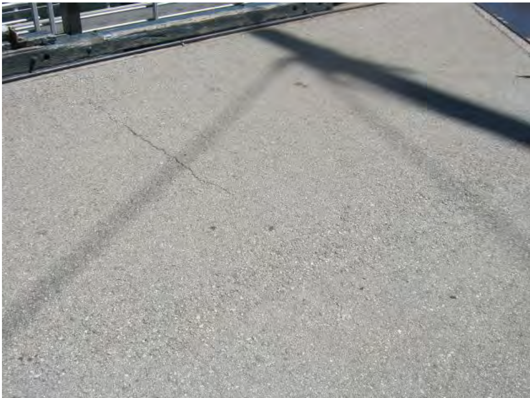
4-Minor Reflective Crack-2011
