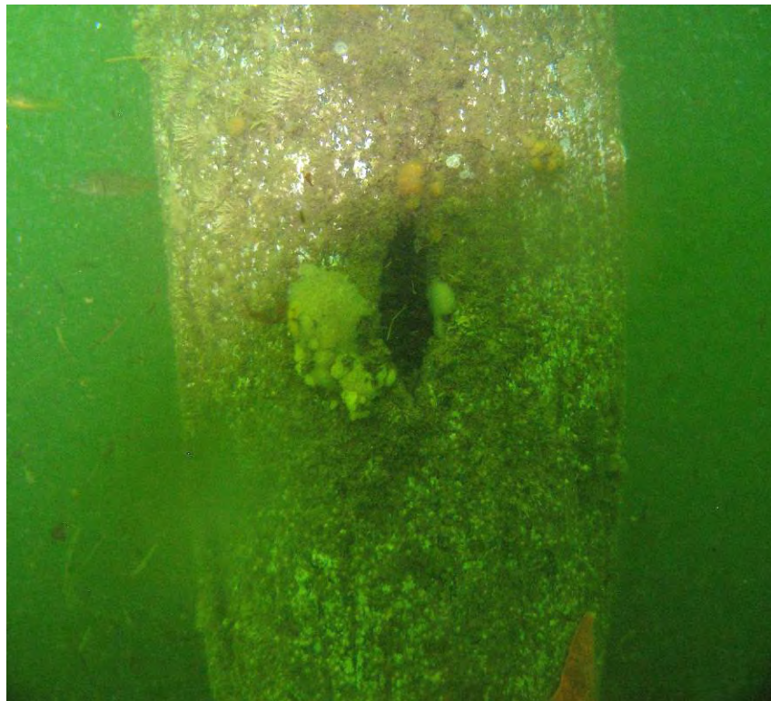
Photo 1-23: Bent 112, Pile 5 - Hole with 30%-80% Section Loss
