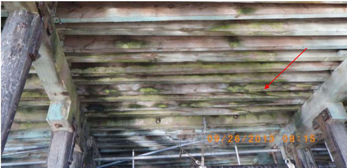
Photo 2-22: Cracks in Stringers on East side of Bents 150-151
