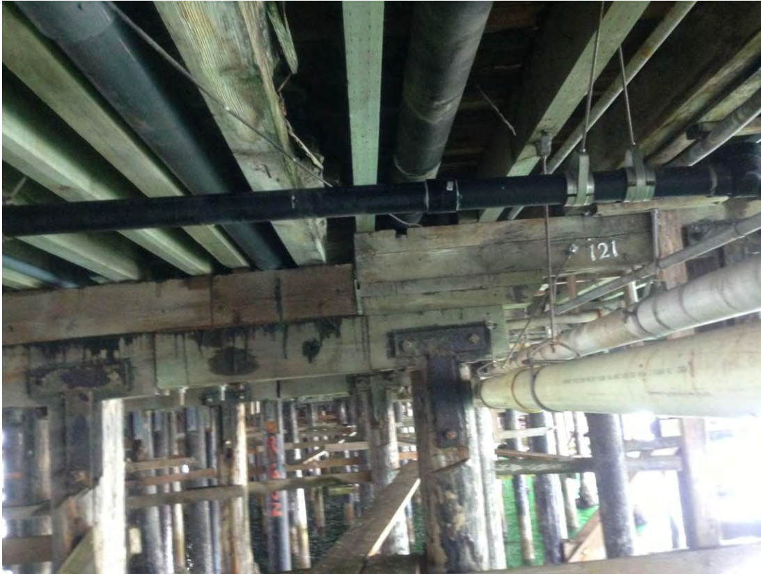
Photo 2-21: Rotten, crushed stringer between Bent 120-121
