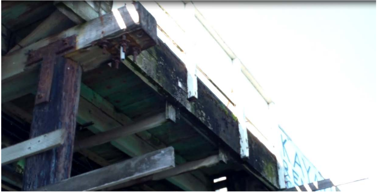
Photo 2-15: Rot on east stringers, Bent 54-55
