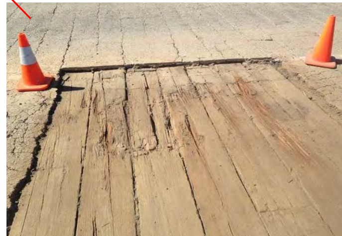
Photo 3-8: Decking with Aligned Butt Joints (near Firefish/ Woodie's)
