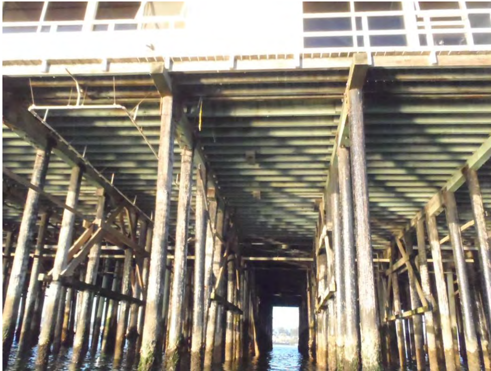
Photo 1-32: Multiple A-frames under Miramar
