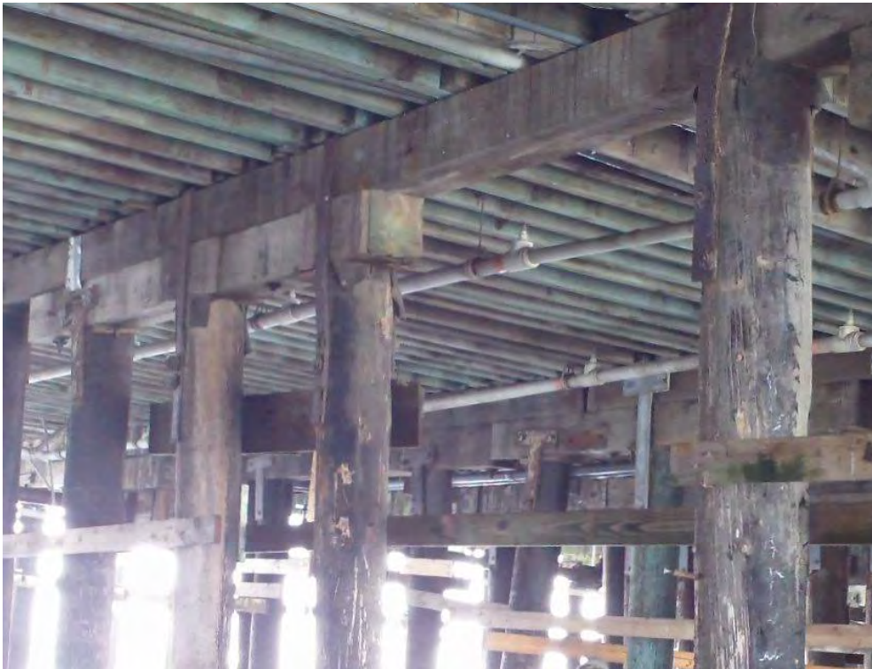
Photo 1-35: U-strap connection (Bent 152)
