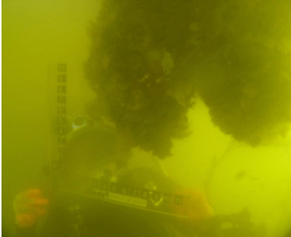
Photo 1-28: Bent 179, Pile 2 – Pile with 100% section loss
