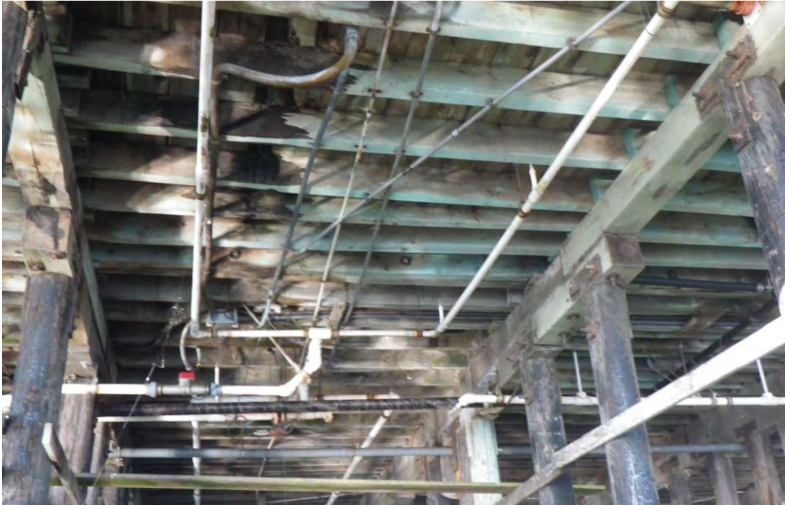
Photo 2-23: Rot between 165-166 (east side)
