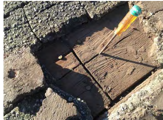
Photo 3-12: Pavement near Miramar (showing loosening nails)
