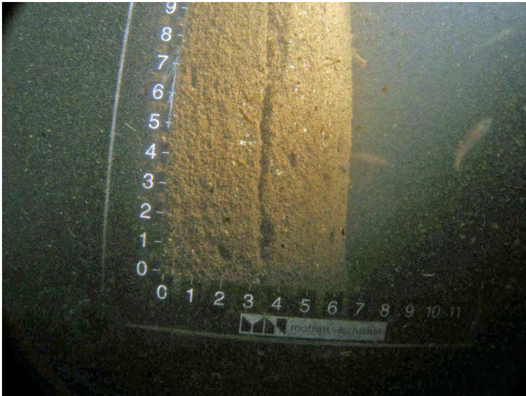
Photo 1-16: Bent 75, Pile 14 – Crack with 5% section loss inside
