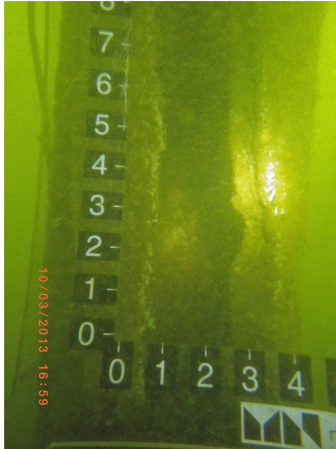
Photo 1-24: Bent 42, Pile 6 – 90% section loss
