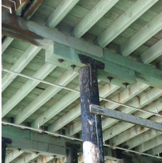
Photo 1-34: Ideal splice cap and T- connection (Bent 122, Pile 2)
