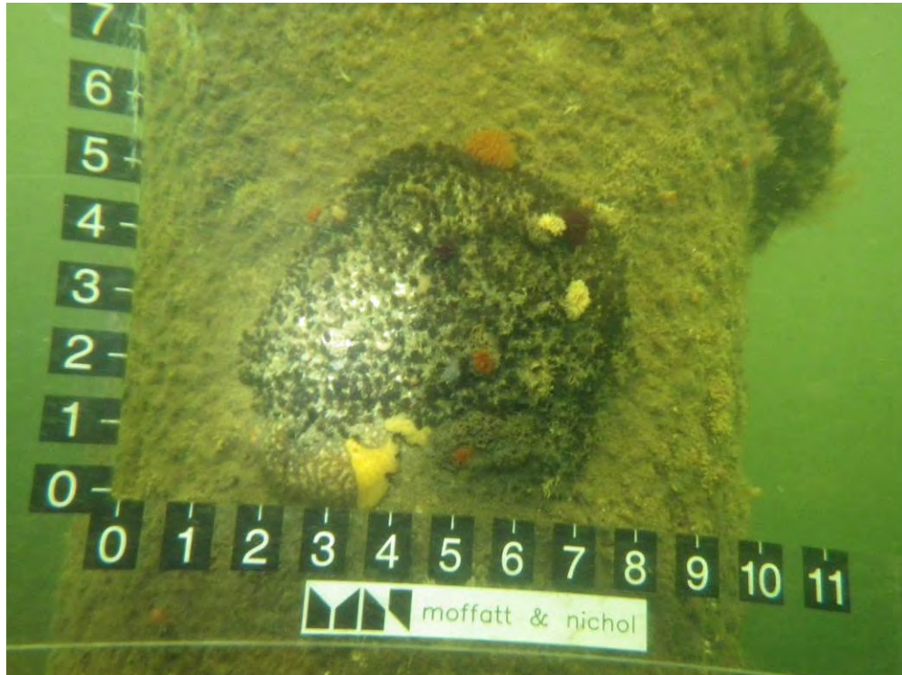
Photo 1-8: Bent 41 pile in excellent condition
