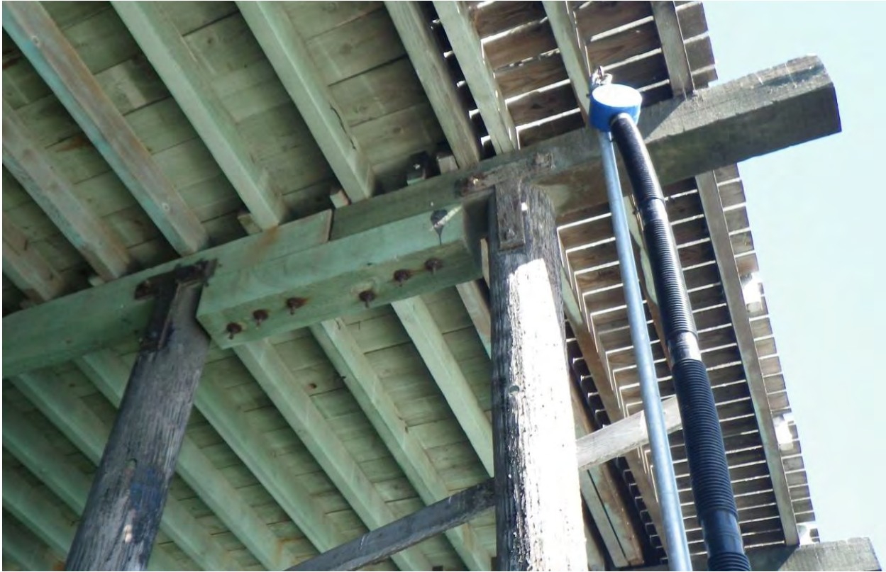
Photo 2-25: Unsupported splice cap (Bent 113, Piles 1-2)
