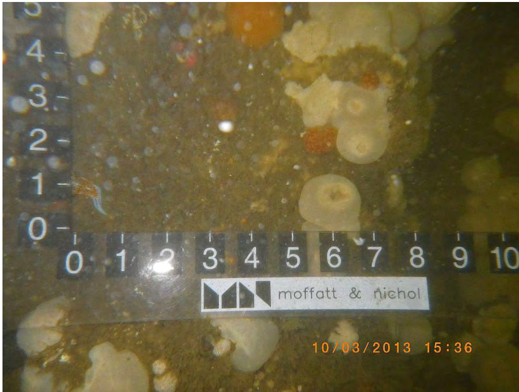
Photo 1-14: Bent 154, Pile in excellent condition
