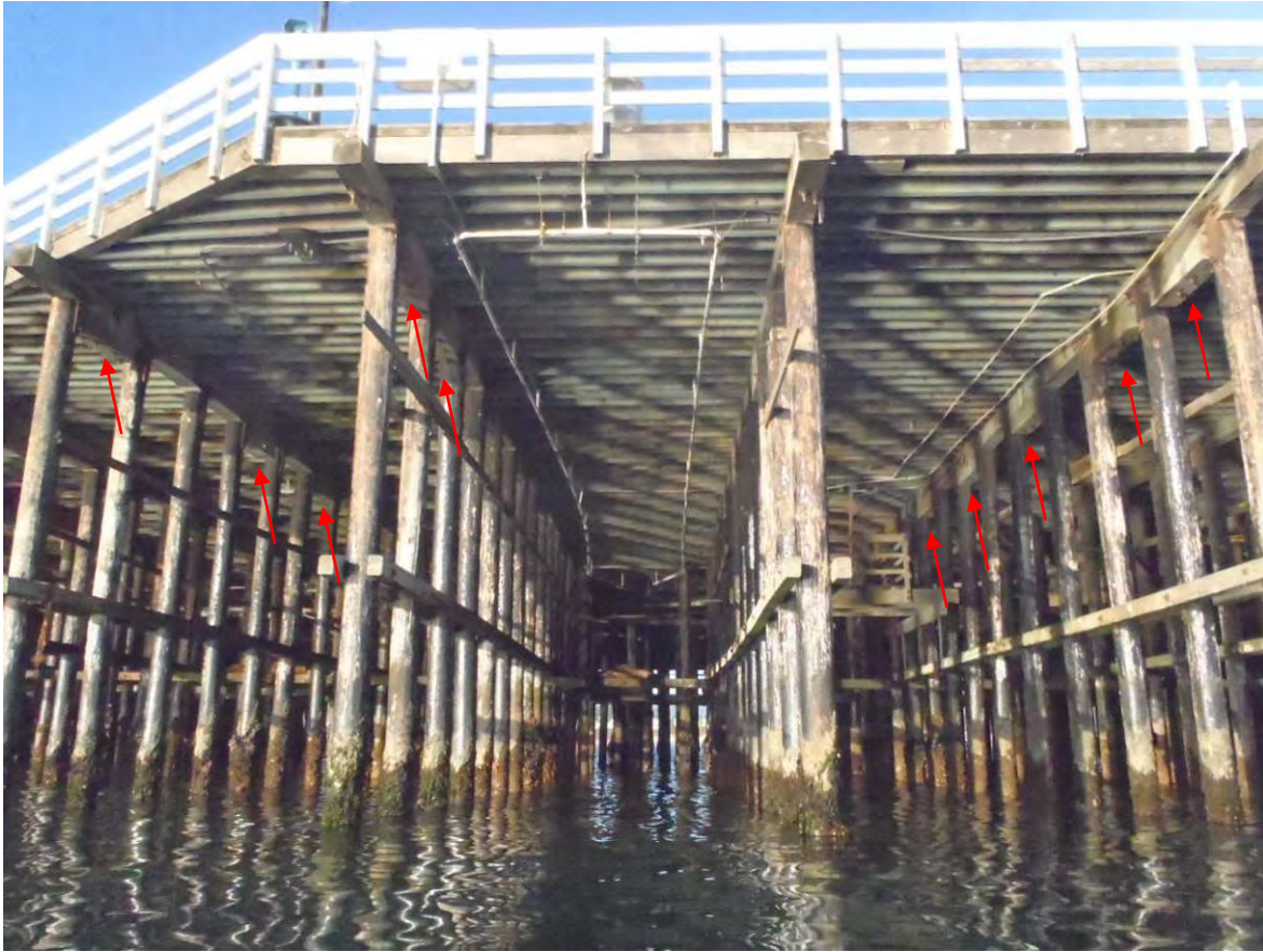
Photo 2-26: Bents 137 – 140 (west side), multiple unsupported cap splices
