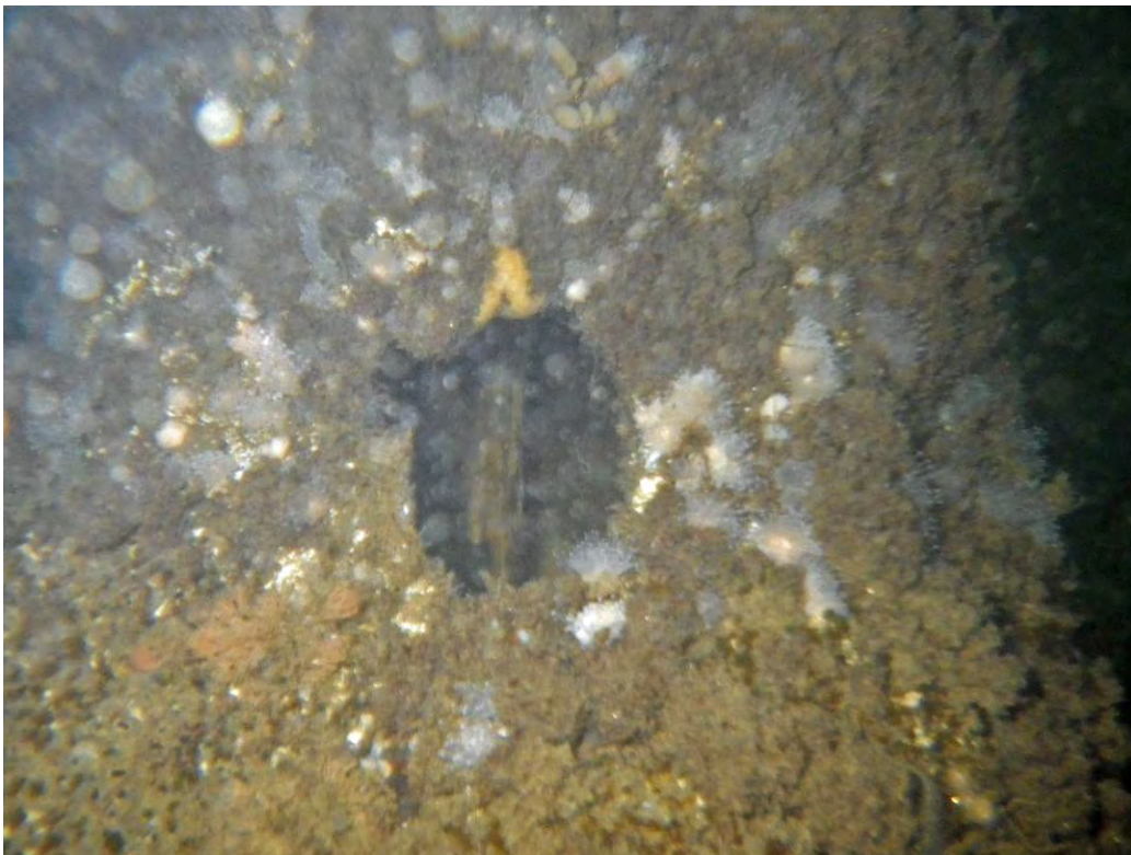
Photo 1-21: Bent 112, Pile 7, Hole with 70% section loss inside
