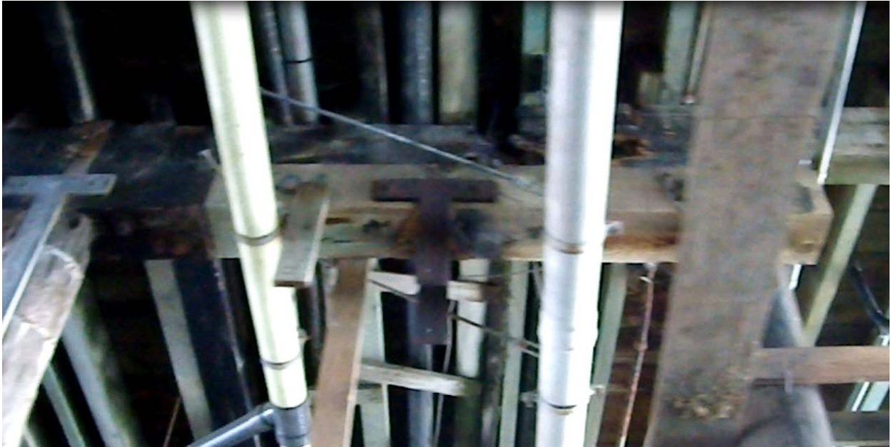
Photo 2-17: Approximate 9 ft. span and fire damage to cap and stringers, Bent 104
