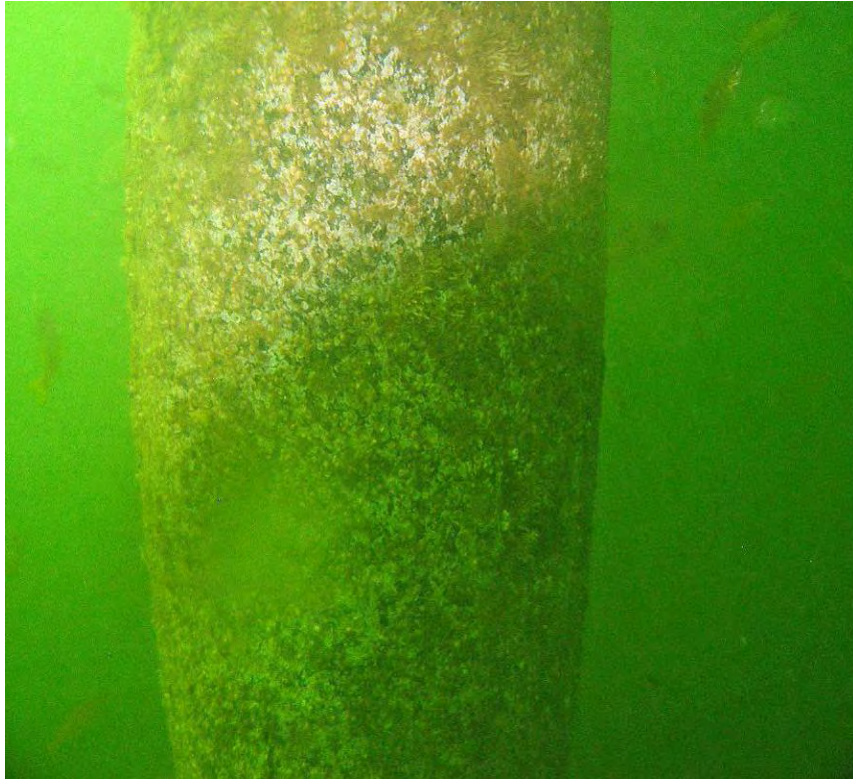
Photo 1-12: Bent 112, Pile 5, portion with excellent condition
