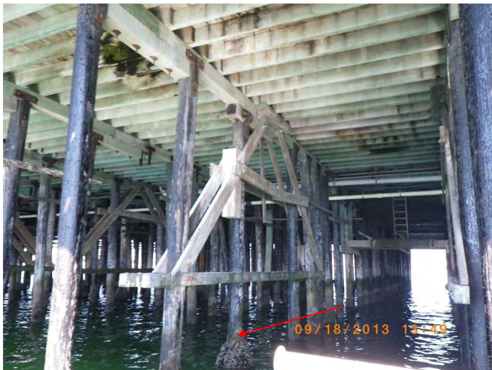
Photo 1-33: A-frame at Bent 119, with damaged pile (see arrow)
