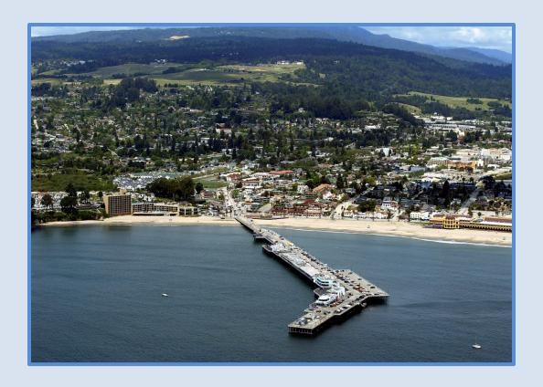
Constructed on a base of over 4,400 Douglas-fir piles, the Santa Cruz Wharf is the longest timber-supported structure in the United States.
