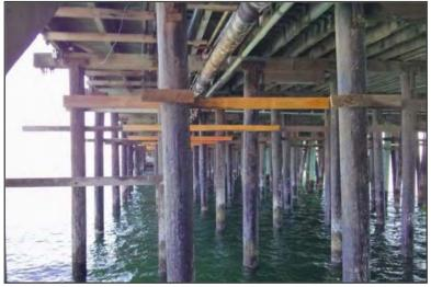
are longer due to water depth at the end. The photo above shows a representative view of the Wharf pile and bent components. On average, 10 to 30 piles are replaced each year. Two inches of asphalt paving overlays the Wharf deck on roads and walkways.
