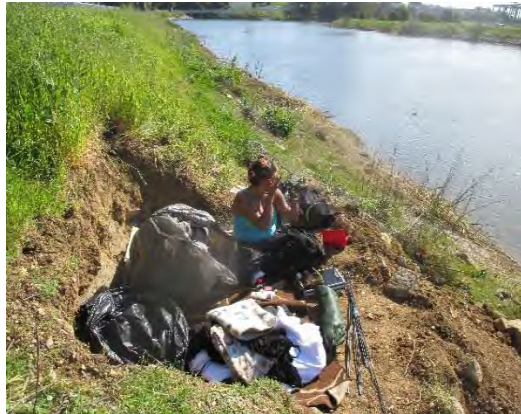
Levee damage caused by illegal camping
